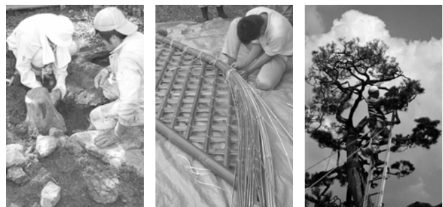
Left) Fig.14 Setting a tsukubai , a stone water basin arrangement Middle) Fig. 15 Making a bamboo fence Right) Fig. 16 Pruning a pine tree
